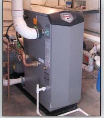
Local installer, Ballard's Plumbing and Heating was contracted to install the Aquas and the installation proved easier than anticipated. First, the Aquas Package took less floor space than the original pool heater. The original metal vent
