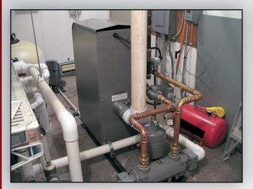
the 399,999 Btu/hr Aquas to replace a pool heater originally firing at 1,000,000 Btu/hr. Due to the high efficiency of the indirect heating method, a lower Btu/hr input boiler could be used. In addition, the 5:1 turndown of the boiler's input rate allowed the XLP to track the heat loss of the pool and modulate the input rate to match the load. Operating at lower input rates reduced operating costs.
